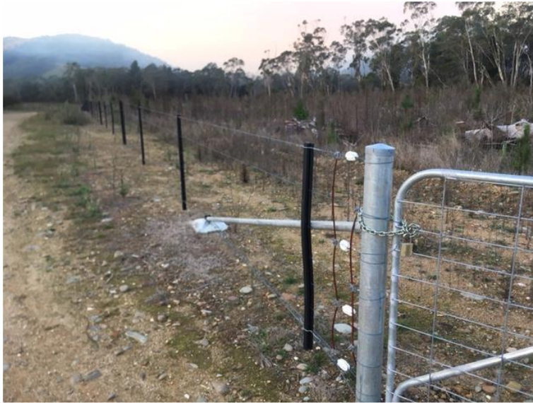
A Gallagher design used to protect a pine plantation. This fence is the conventional fence height of around 1.2 metres only but the induction effect deters animals. Upper Ovens Valley Landcare
