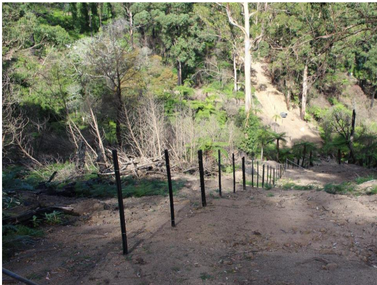
Electric fence installed in steep and rough country utilising less materials for handling than conventional fencing. Gallagher
